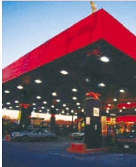
The demand for fuel at high volume stations depends on several demographic variables. Morning and evening rush hours, and lunch, are peak operating times.
