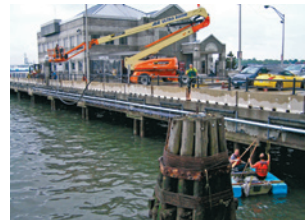
Final attachment of the pipe to the pier
