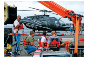
Installation work during ongoing helicopter traffic
